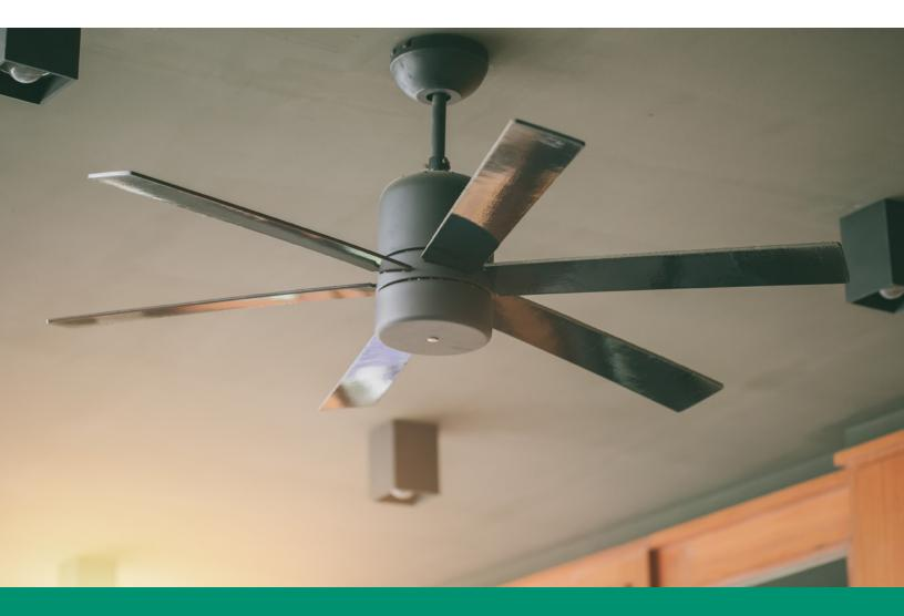
When moving this direction, the tilted blade edges cut through the air, pulling cool air up to displace and push down the warmer air near the ceiling.
