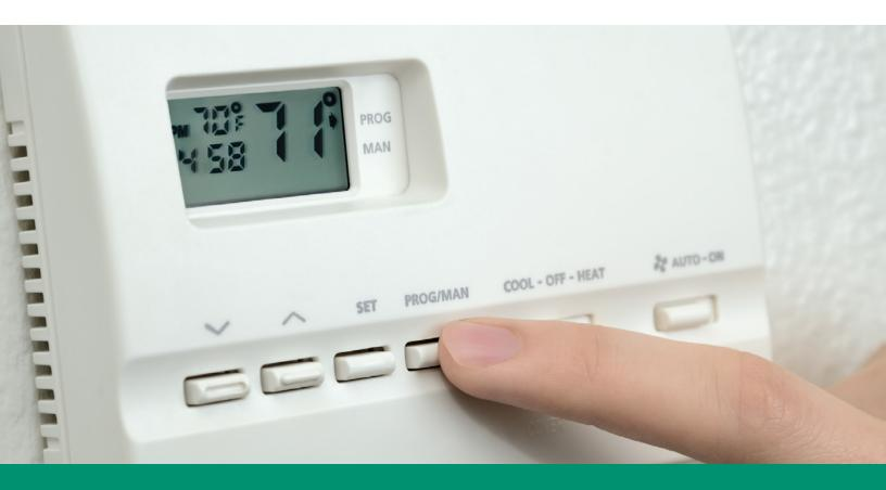
By adjusting the thermostat lower by just 7 degrees overnight, you could <u>save up to 10%</u> on your heating cost annually.
